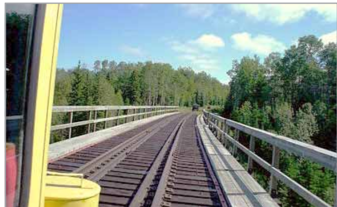
Cash Creek Trestle.
