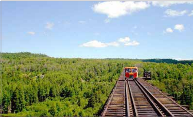
Pass Lake Trestle (aka Blende River Viaduct).
