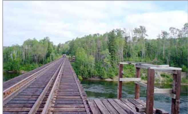
Nipigon River Trestle.
